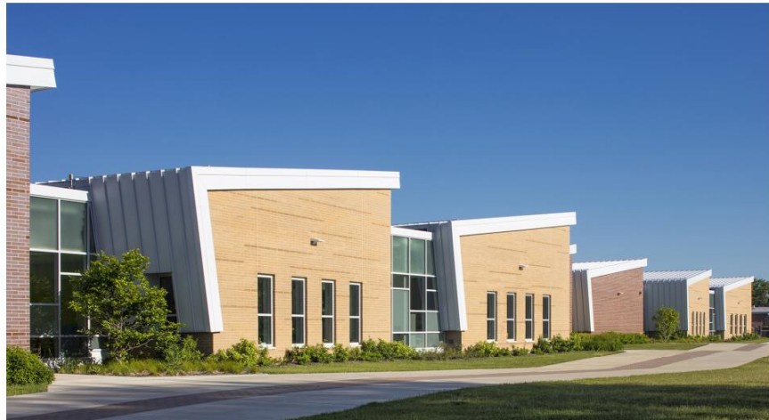
■ Classroom bars along the east façade feature playful brick patterns and metal roofs that slope down to become walls.
