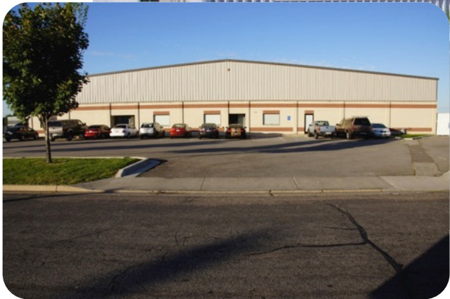
Before and After Exterior
