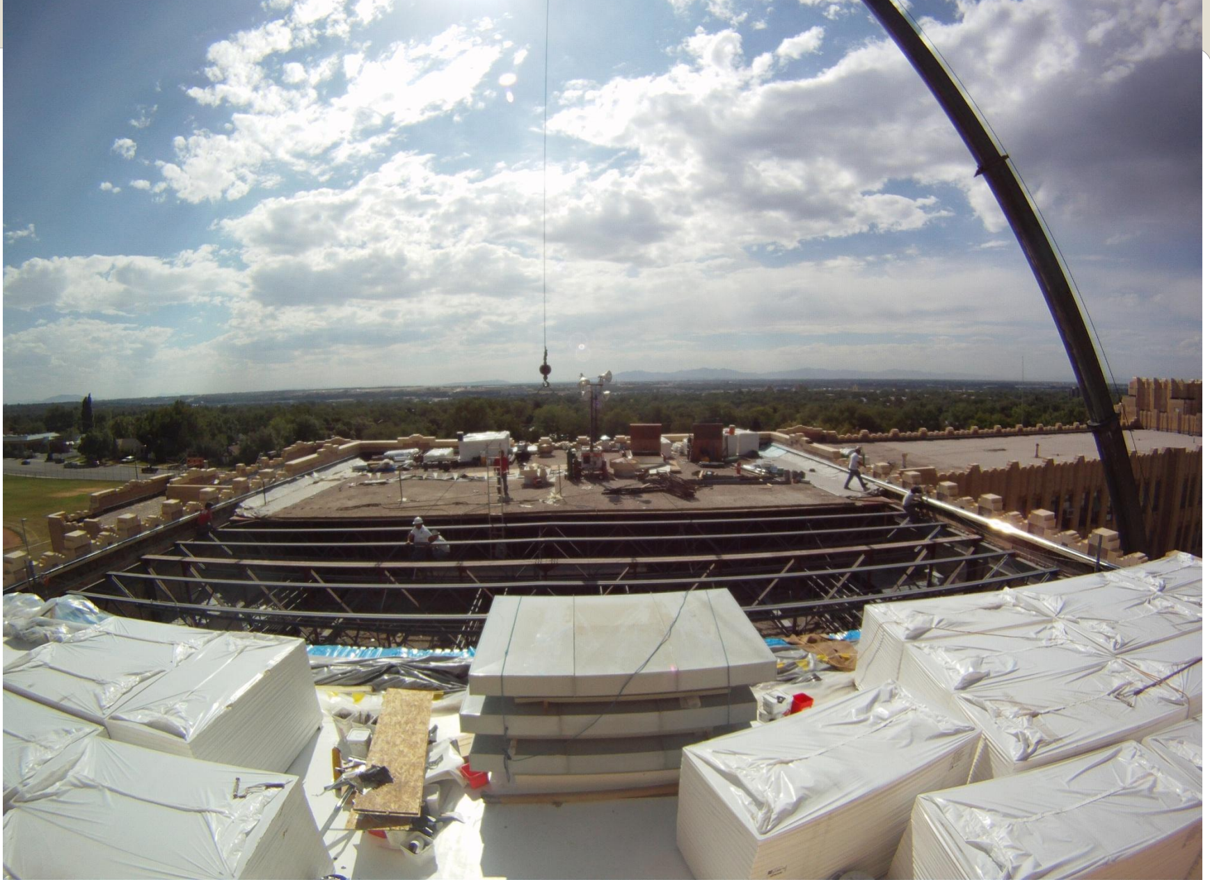
Photo Caption: We replaced the roof in 32-hour segments to protect the ceiling beneath
