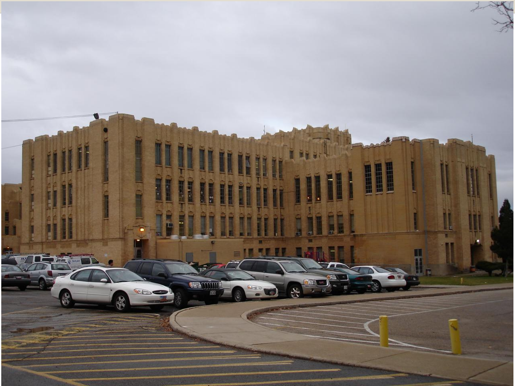
Photo Caption: Before the renovation the walls were dangerously lacking in reinforcement
