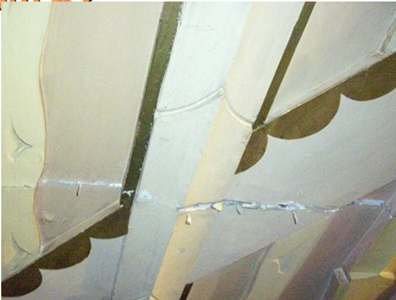
Photo Caption: The plasterwork was faded and badly damaged
