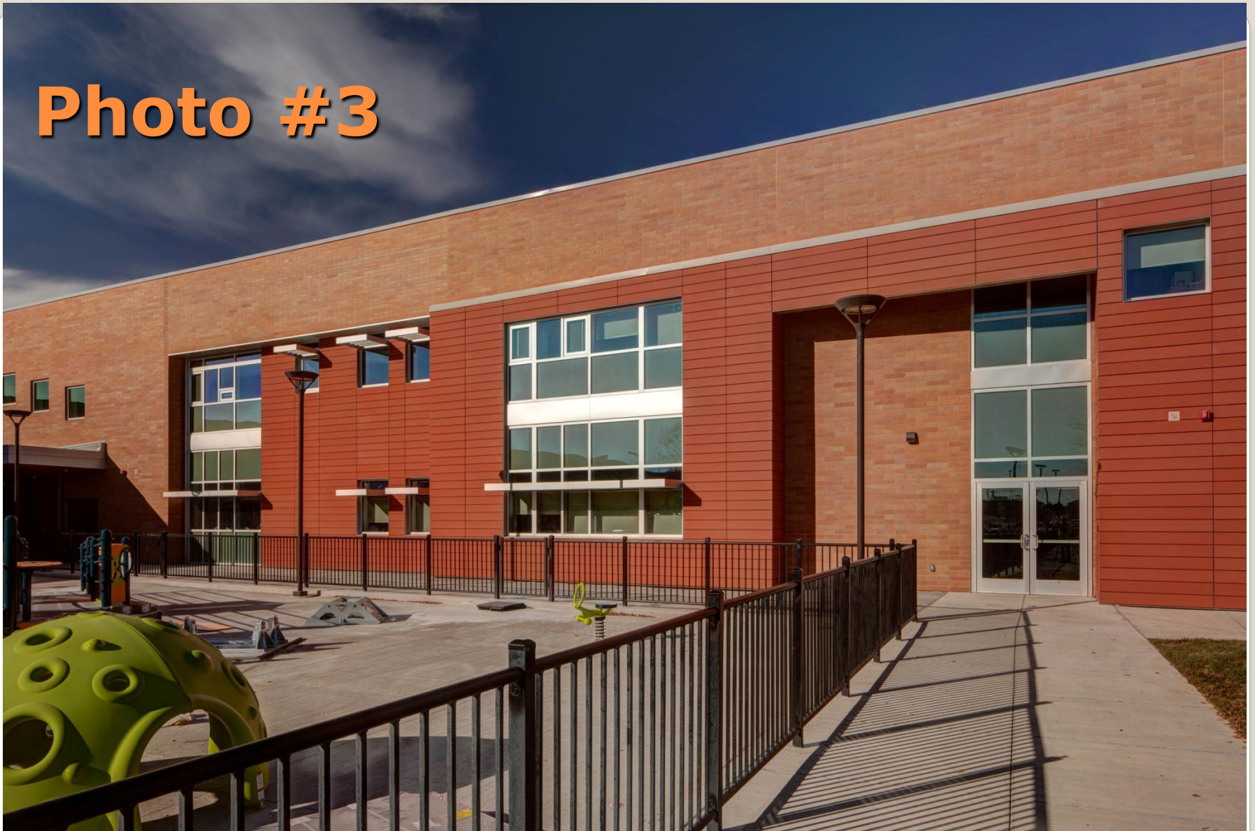
Hartvigsen K-12 Special Needs School – Exterior interactive playground area
