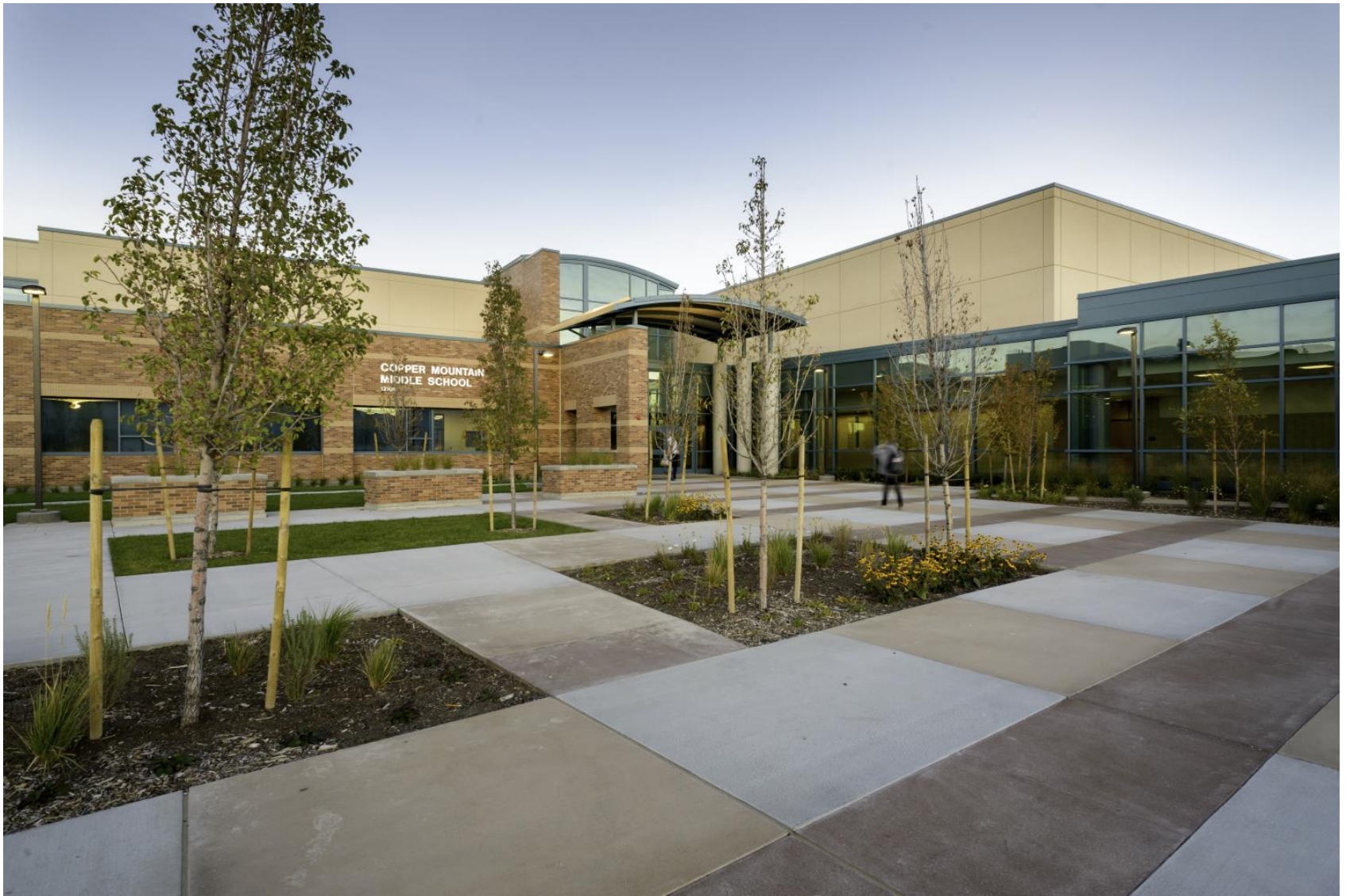
East Facing Main Entry and Courtyard
