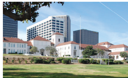
Existing Photo: View from Moreno Drive
