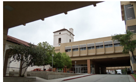
Existing Photo: Bridge between Building A and B1
