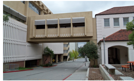
Existing Photo: Bridge between Building A and B2
