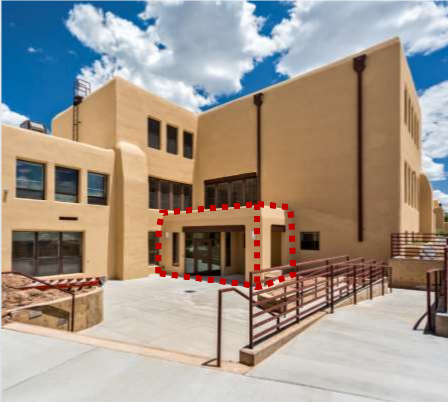
Rear Basement Vestibule Addition
