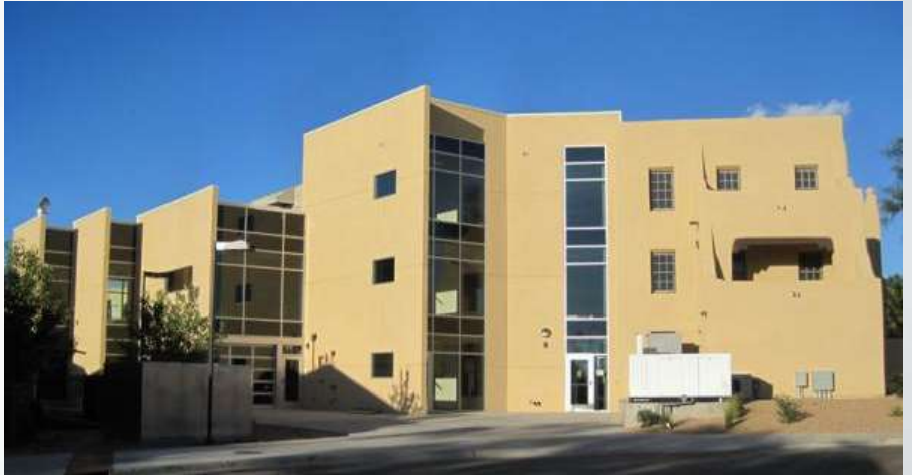
NMSD Connor Hall, SSWA
