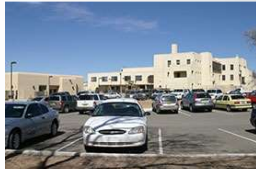
Side view of Connor Hall, 2009
