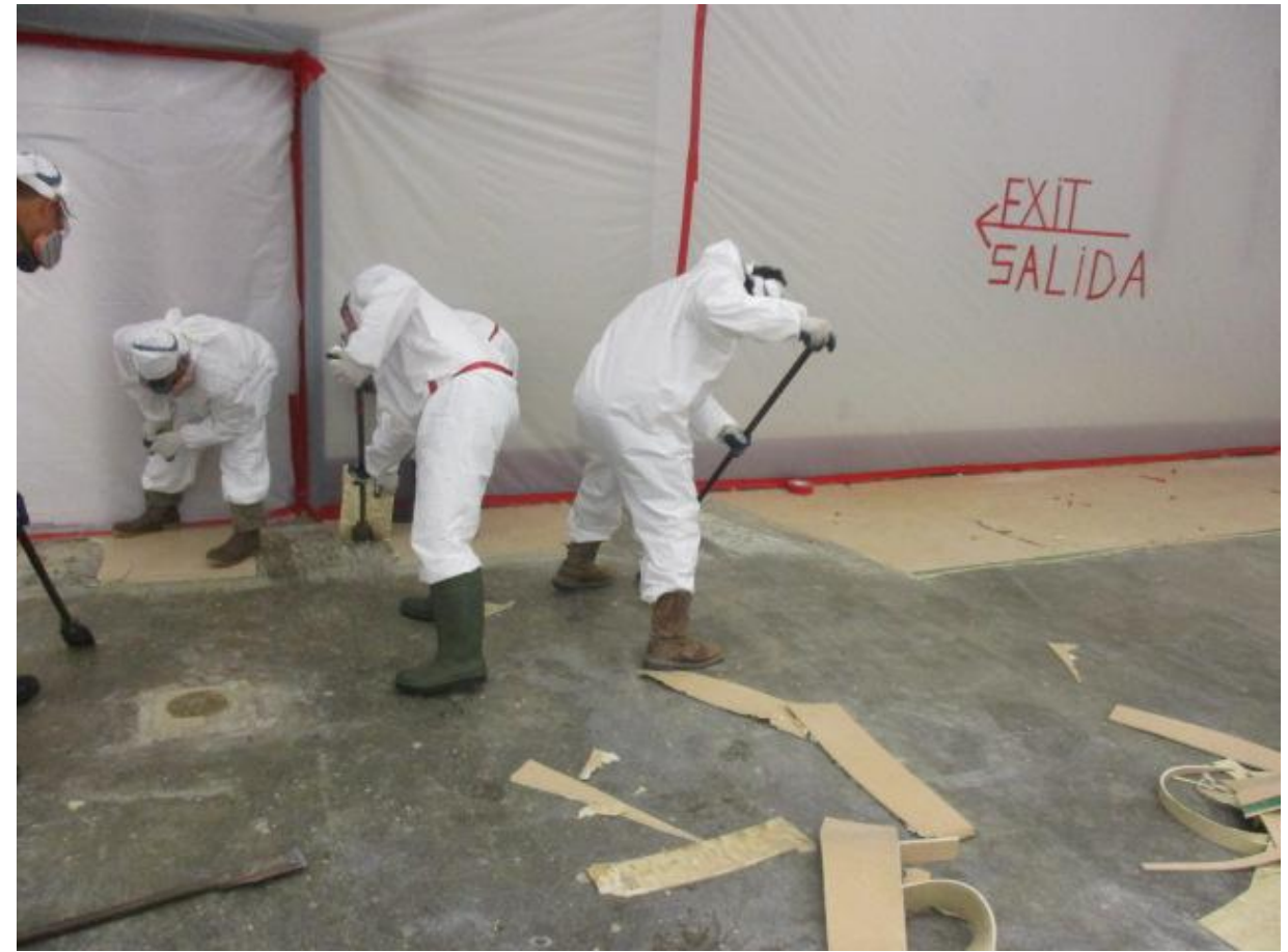
Flooring material removal with machine and by hand.
