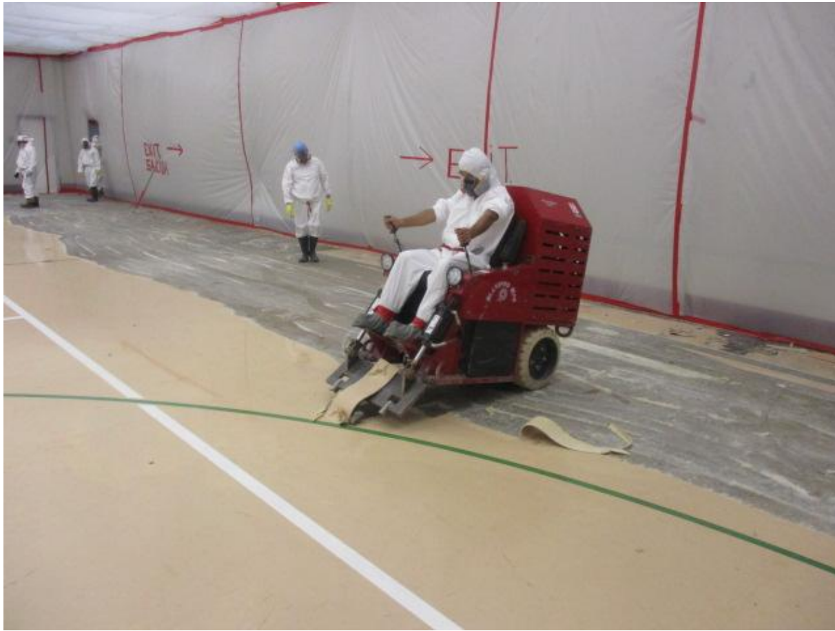
Flooring removal with floor tile removal machine.
