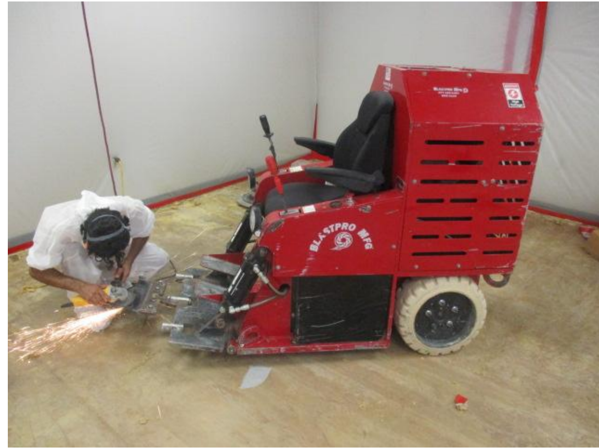
Flooring removal with floor tile removal machine.
