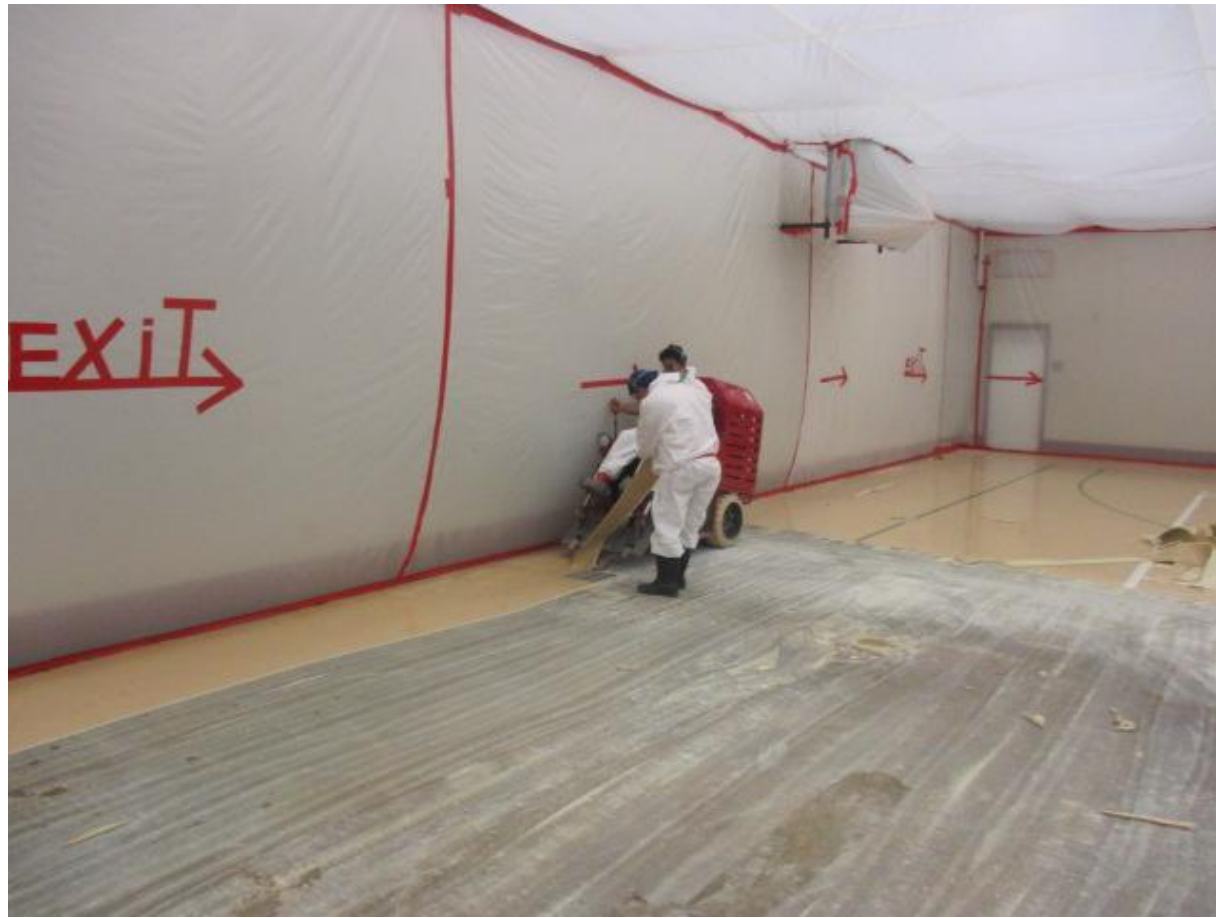
Flooring material removal with machine and by hand.
