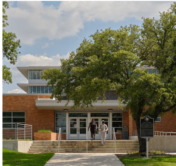
Historic entry of new build
