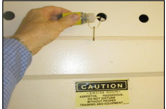
Check Air flow at critical areas
