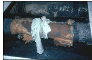
REPAIR WATER LEAKS
