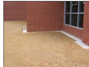
Slope Away from Building
