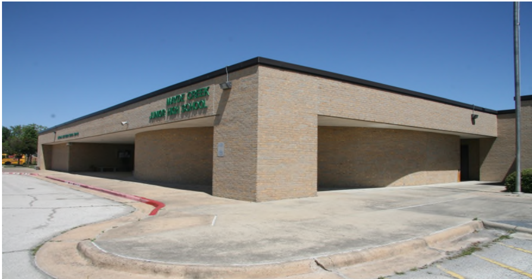
Existing Condition – Main Entry Mayde Creek Junior High School
