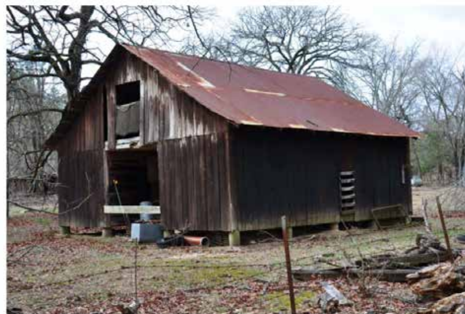
Typical Transverse-crib Barn , Swink vicinity, Choctaw County (023-A). This typical example in the Ouachita foothills contains the three diagnostic traits identified by Jordan-Bychkov of: (a) stalls, (b) grain bins, and (c) hayloft, as well as a tack room. The central runway remains in use for storage, with a single board to deter wandering cattle.
