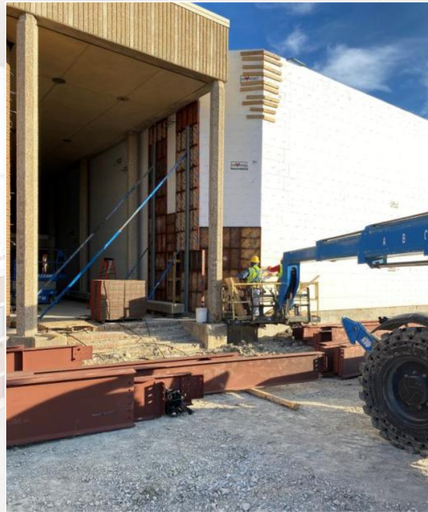
Storm Shelter Tie-in to Existing Building
