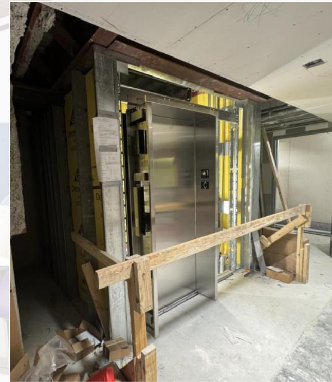
Elevator Installation to Existing Building
