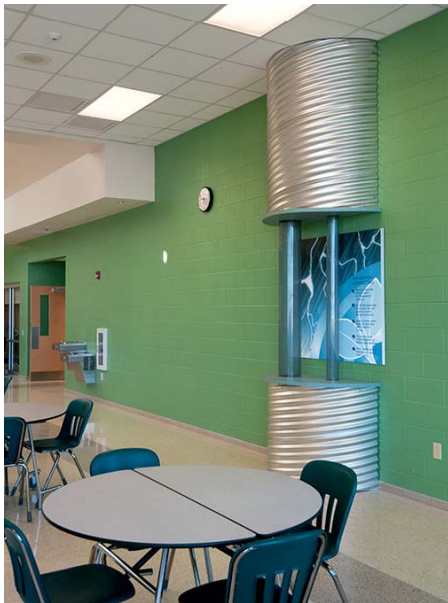
Exposing building systems, such as clear pipe rain leaders shown above, provide an example of using the building as a teaching tool.
