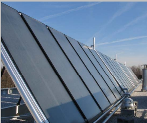
ROOF MOUNTED SOLAR PANELS
