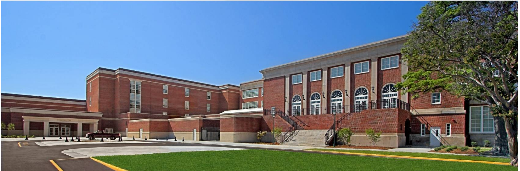
RENOVATED AUDITORIUM ENTRY
