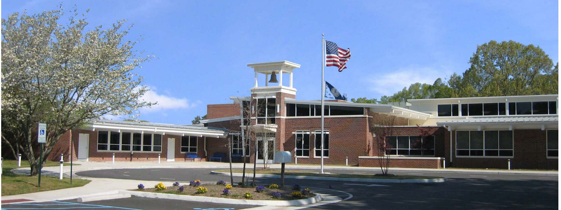
Abingdon Elementary School Additions & Renovations
