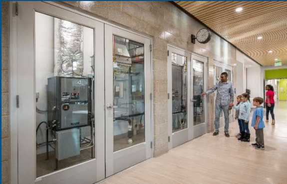
Exposing mechanical systems
