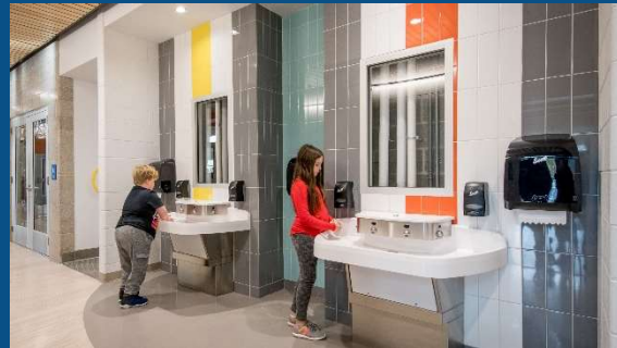
Exposing plumbing systems
