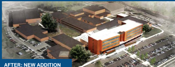
AFTER: NEW ADDITION
