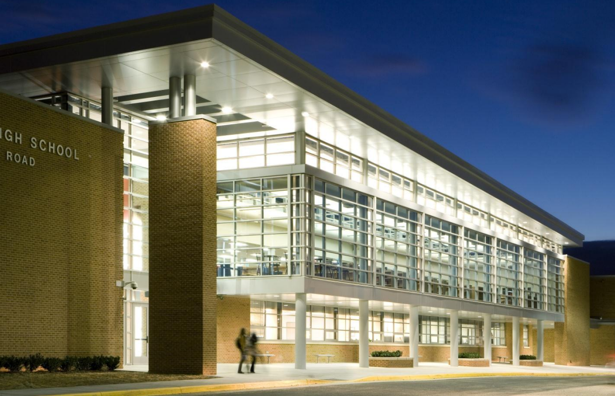
STREET PRESENCE: Main Entrance - After
