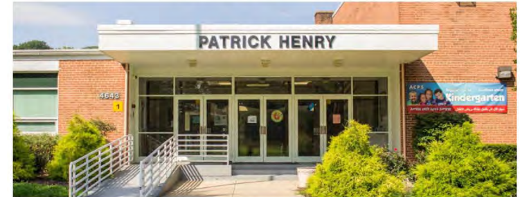
At this point, demolition of the old Patrick Henry school facility has been suspended until early April while all considerations are being explored. The old recreation center will still be demolished to provide a proper flow between the old and new school buildings. (Courtesy photo)
