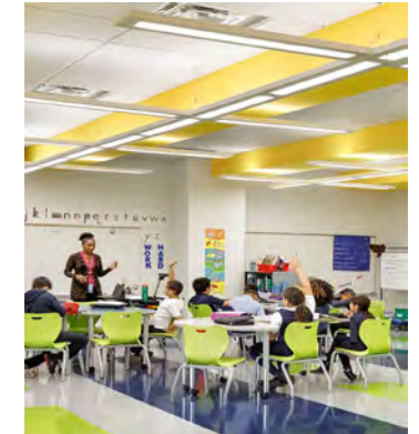
energy efficient lighting
