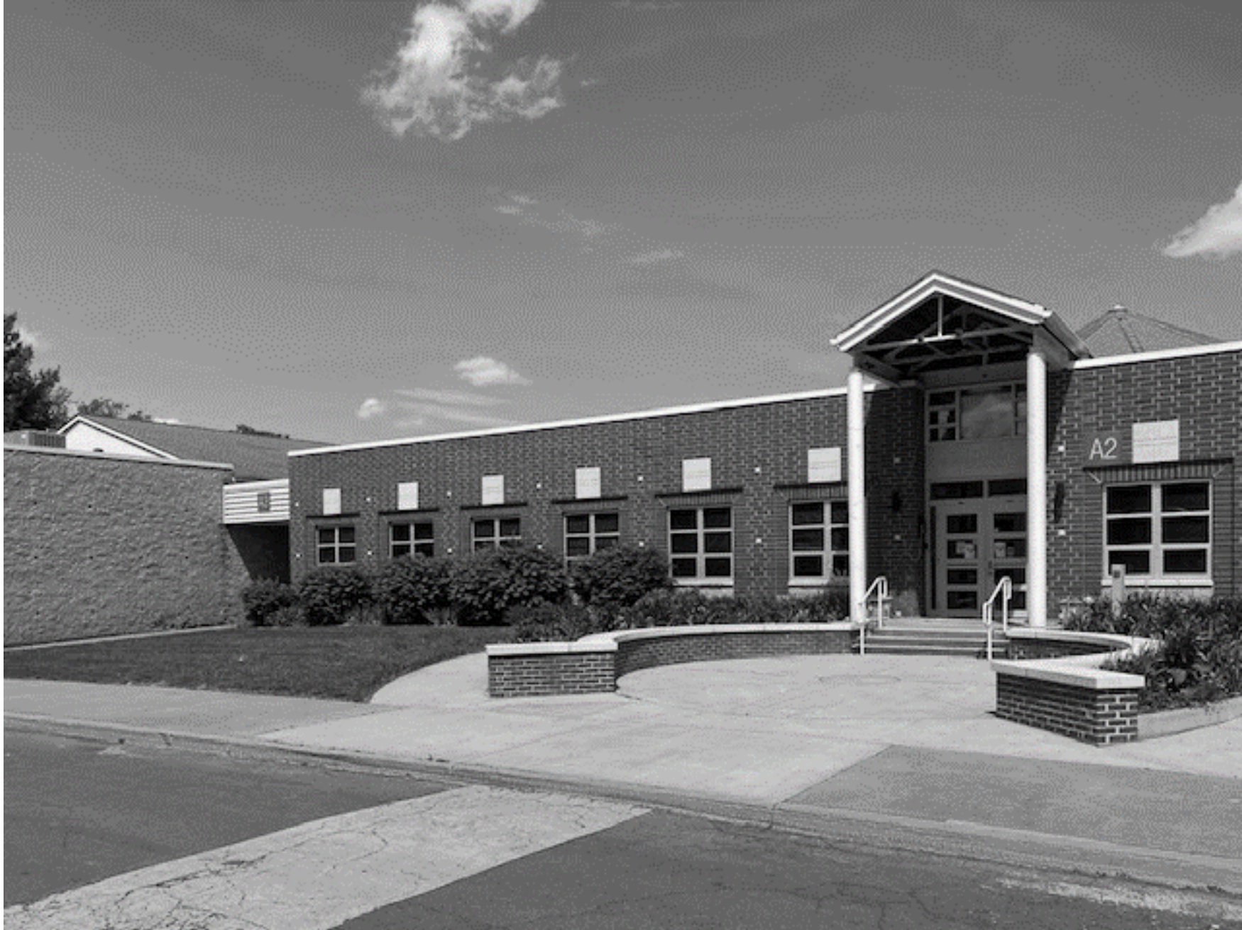
Front Entry from West - Before
