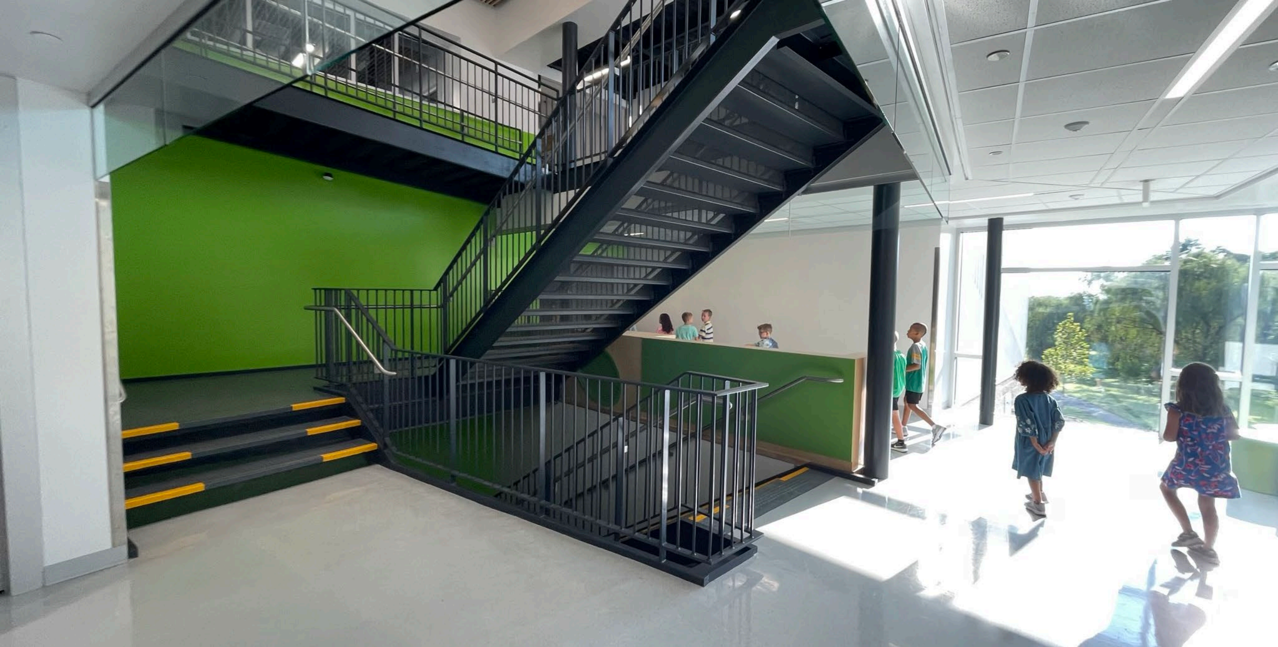
Open Stair @ New Learning Wing
