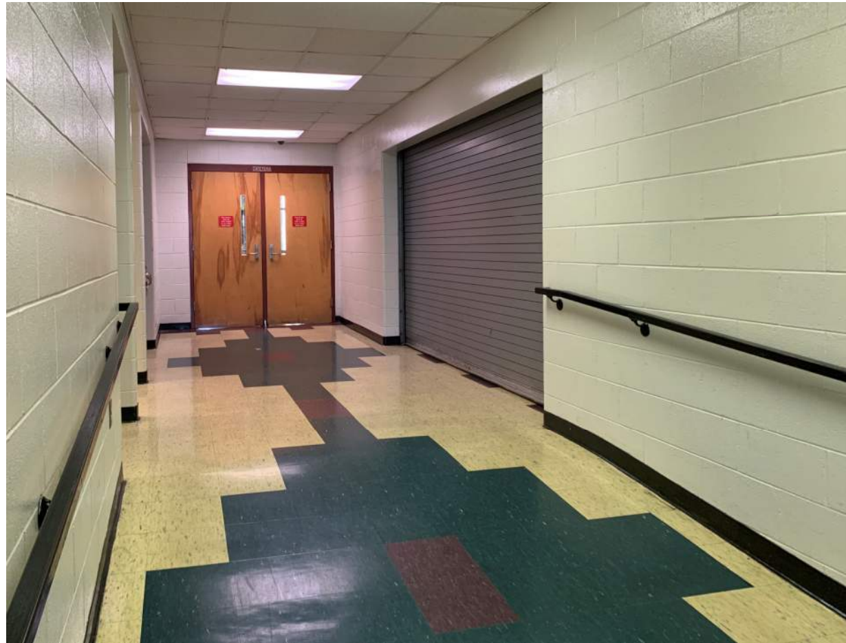
Renovated in Place
