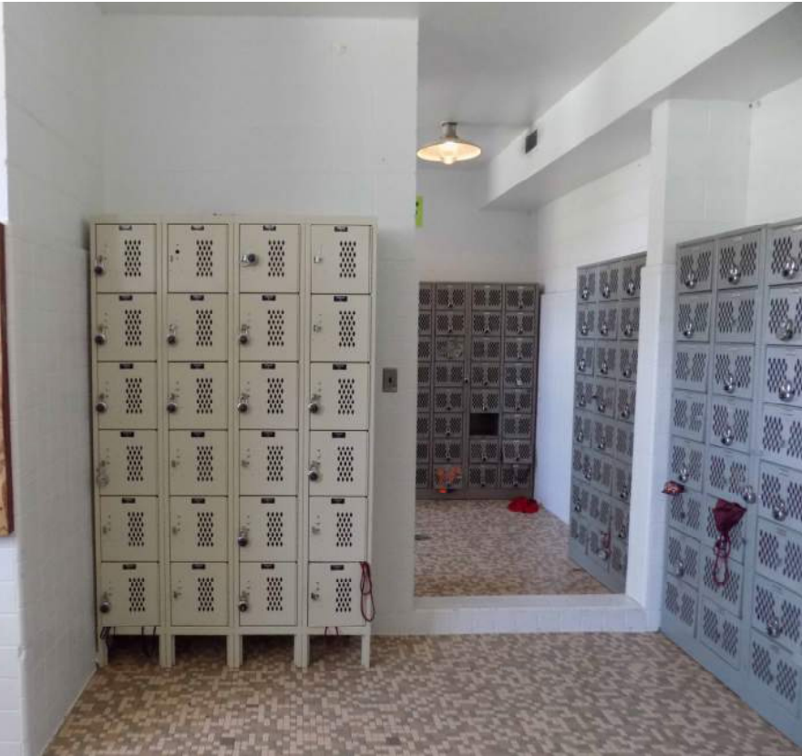
Existing 1960's Wing
