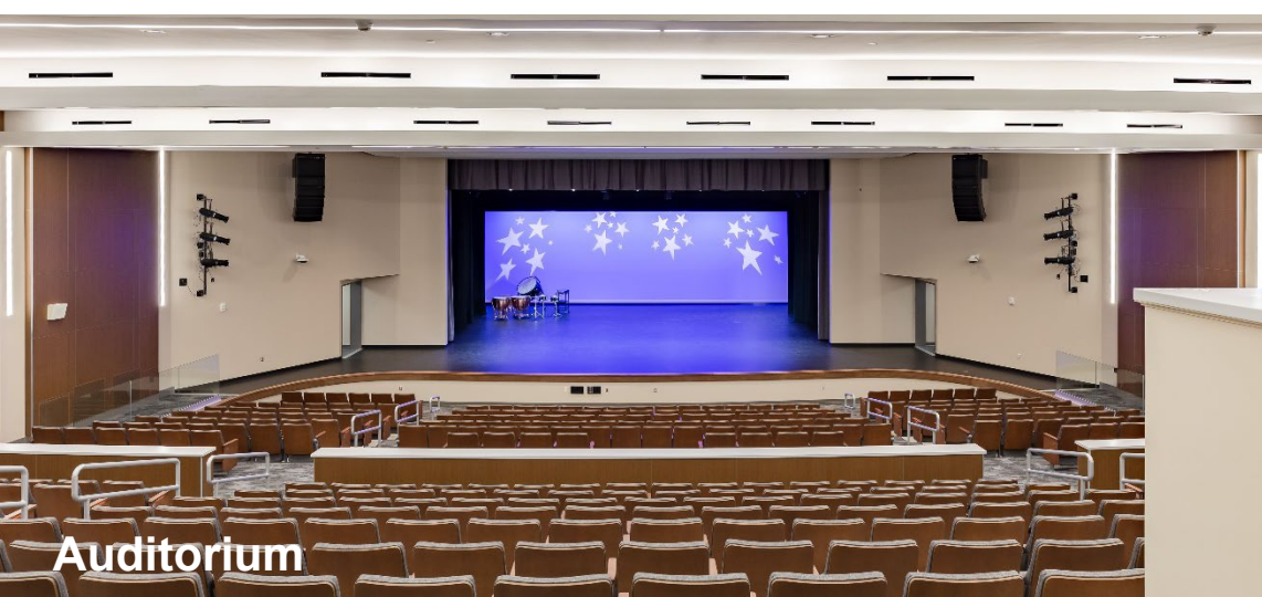
Auditorium – Theatrical Rigging
