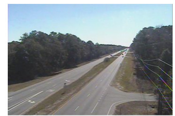
Hwy 21 / Clarendon Road 2768 TRASK PARKWAY
