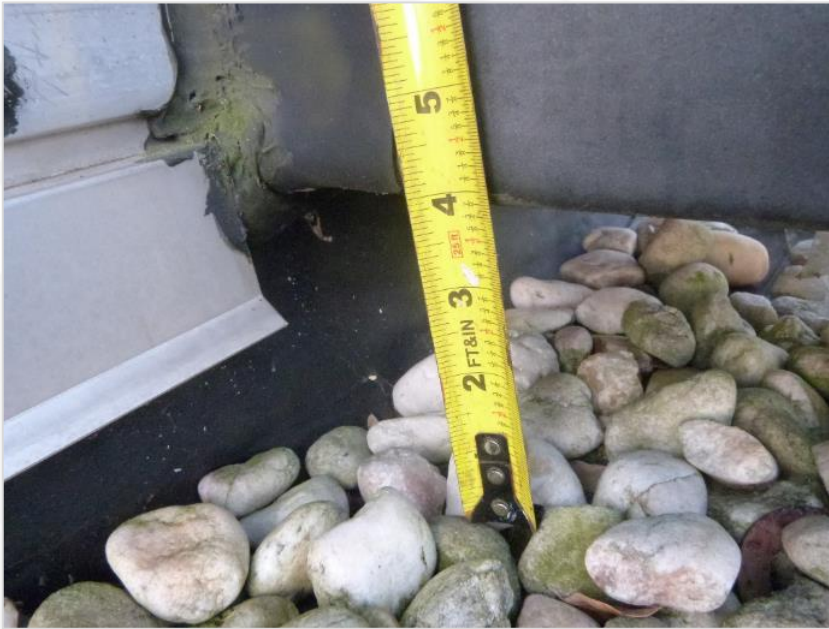
2" Flashing @ Window Interface (Old Roof)
