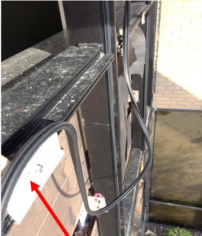
Temporary glazing retainer clip ready to receive new glass
