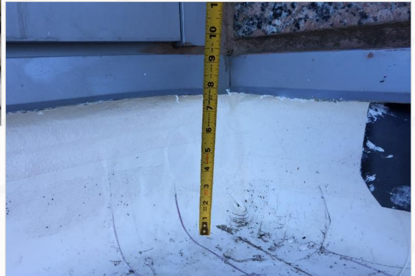
New Roof 8" Flashing
