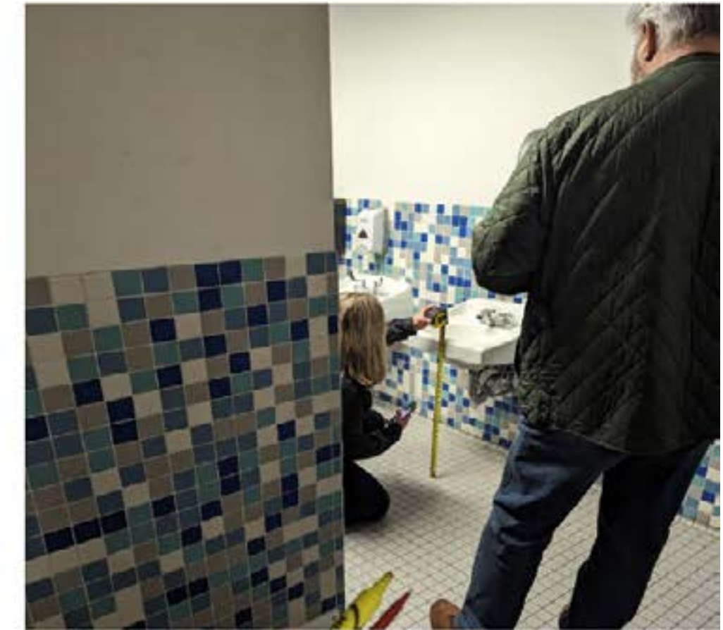
Measuring lavatory rim height and knee clearance at Beverly Elementary
