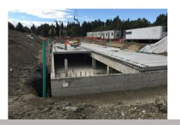
A 56,000 cubic foot detention vault capture stormwater from hard surfaces and building roofs.
