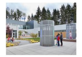
A mechanical room below the second floor courtyard helps balance cut and fill on site. The perforated metal shrouds around the roof hoods in the courtyard are lit with LED lights that change color as the hood draws in fresh air and exhales exhaust air.
