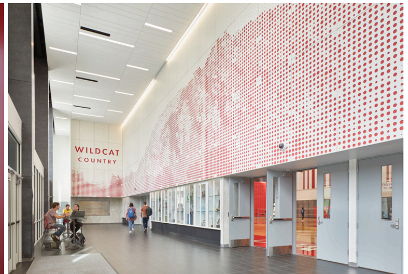
Custom fabricated perforated panels in the gym lobby reflect an abstracted Mount Si image and provide acoustic absorption.
