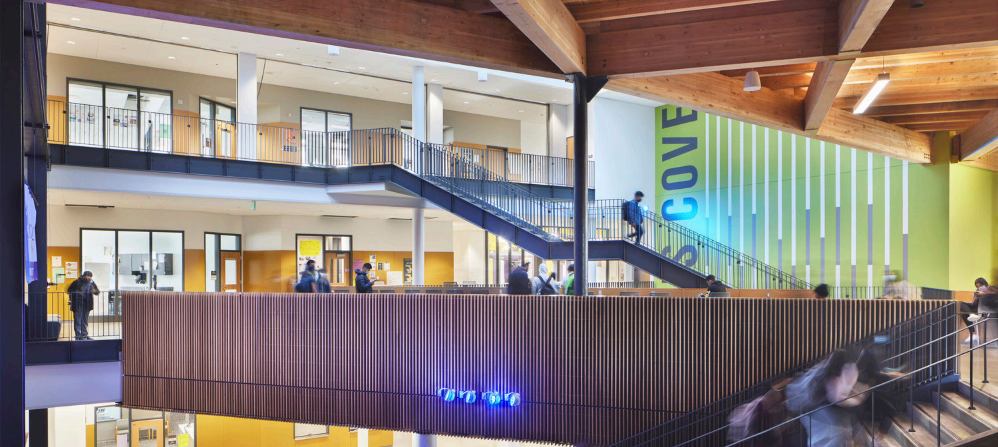
The commons features timber framing with glue-laminated columns and beams; wood decking, and purlins for a biophilic approach to structure that reduces embodied carbon
