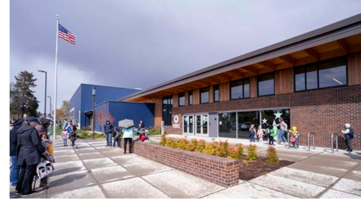
The entrance to Birney is next to the Family Connection Center (just inside the windows) creating a welcoming experience for students, parents and community partners.
