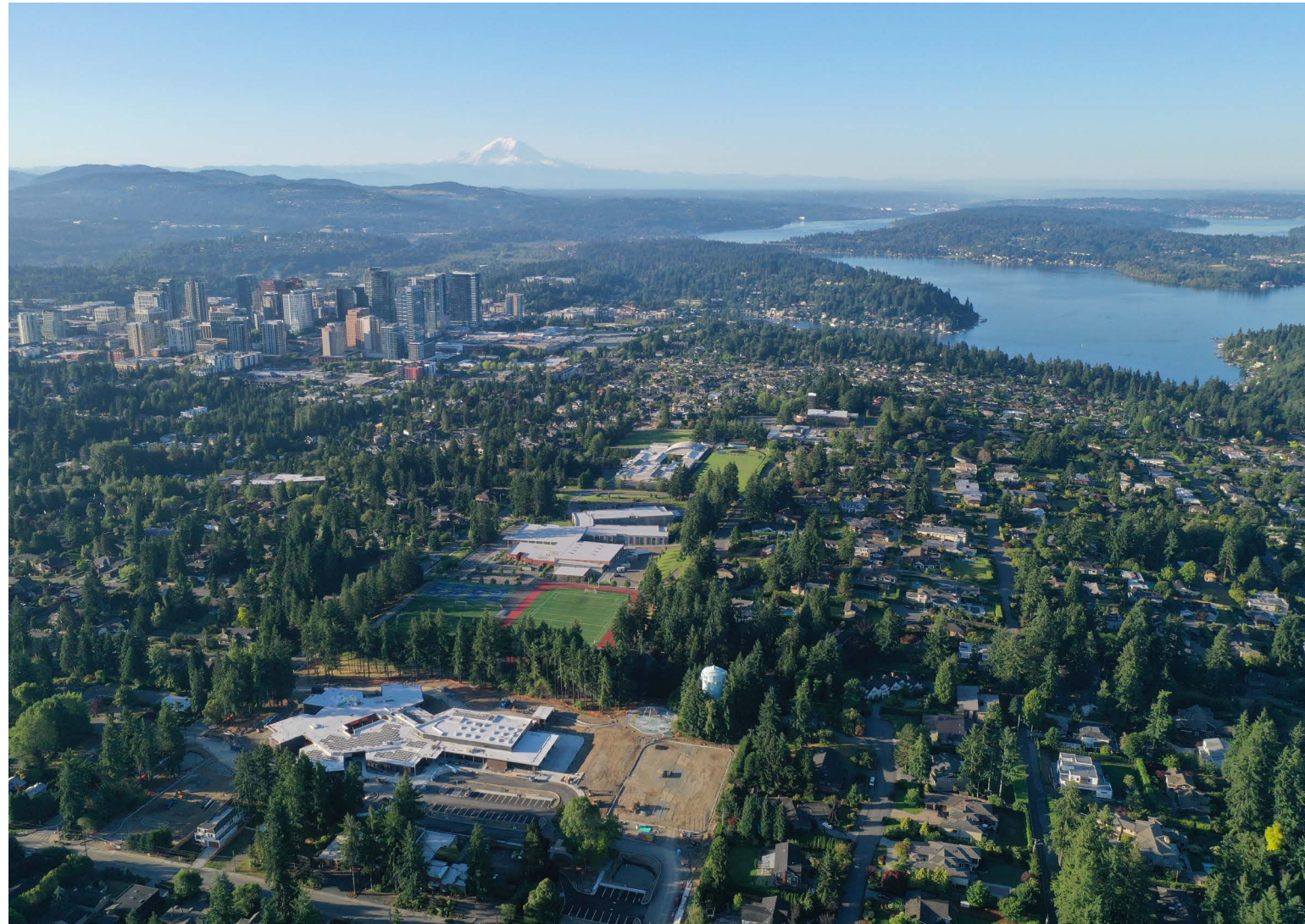
Clyde Hill Elementary School sits on the Clyde Hill ridge, a part of a series of schools and civic buildings surrounded by evergreens and a residential neighborhood with dramatic views of the skylines of Bellevue and Seattle and the Cascade Mountains.
