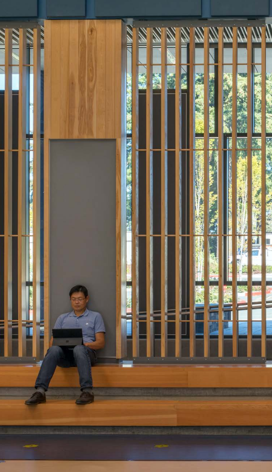
Wood screens filter light and views from the commons to the school's "front porch." Tiered wood seating was created from trees selectively harvested from the site.
