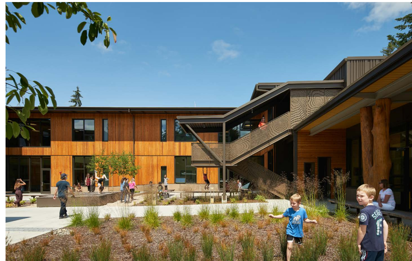
Above—STEM classroom indoor-outdoor connections
