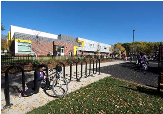
South Facing Playground and Childcare Center
