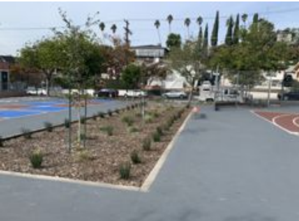
STORM WATER RETENTION
