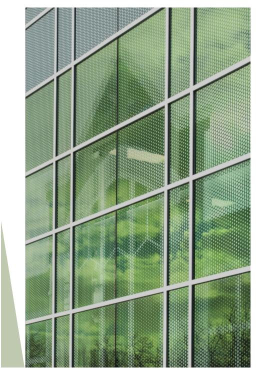
A ceramic frit screen with the historic facade pattern was incorporated into the gymnasium glazing system with the dual purpose of controlling solar heat gain while acting as a reminder of what came before.
