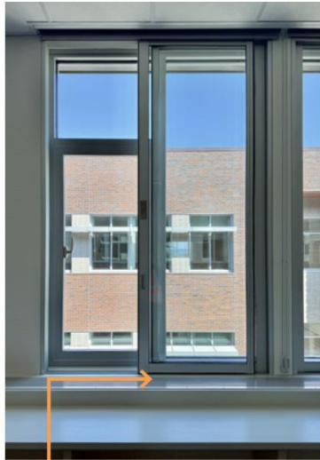
Slide sound barrier window open to access exterior operable window
