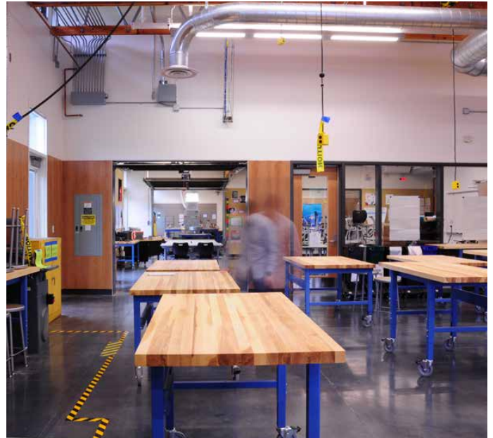
High bay space in the large Fabrication Lab with clerestory daylighting, overhead power distribution and direct connections to the clean tech room.
