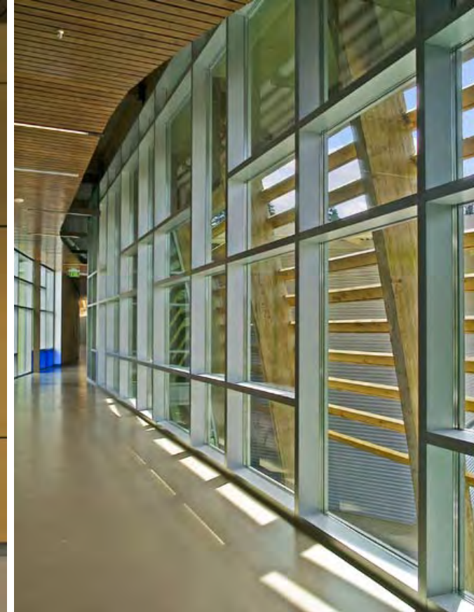
"Truth" wall: Building systems are exposed from the main hallway. The path of light through sunshading elements educates occupants about time and seasons.
