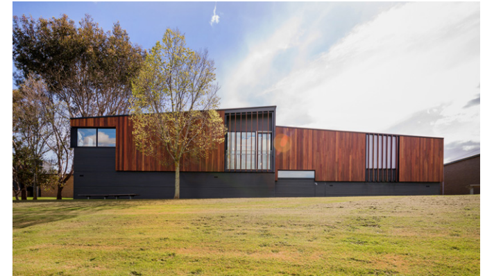
The Learning Project: designed not to look like a relocatable building
