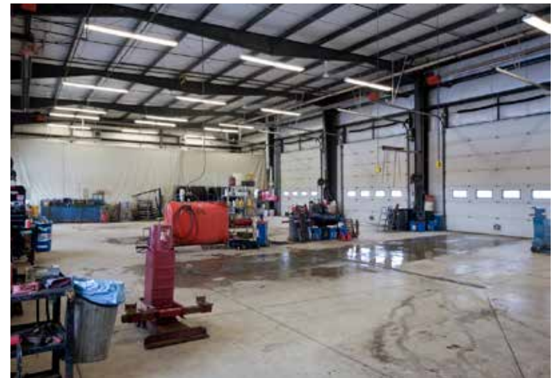
Clockwise from top left: learning quad; science park; bus maintenance facility
