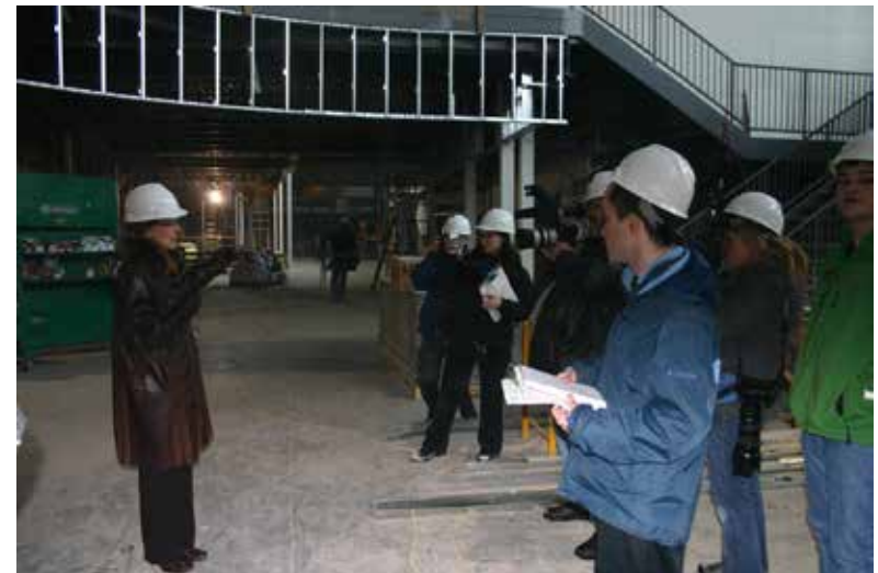
Touring staff and media during construction.
