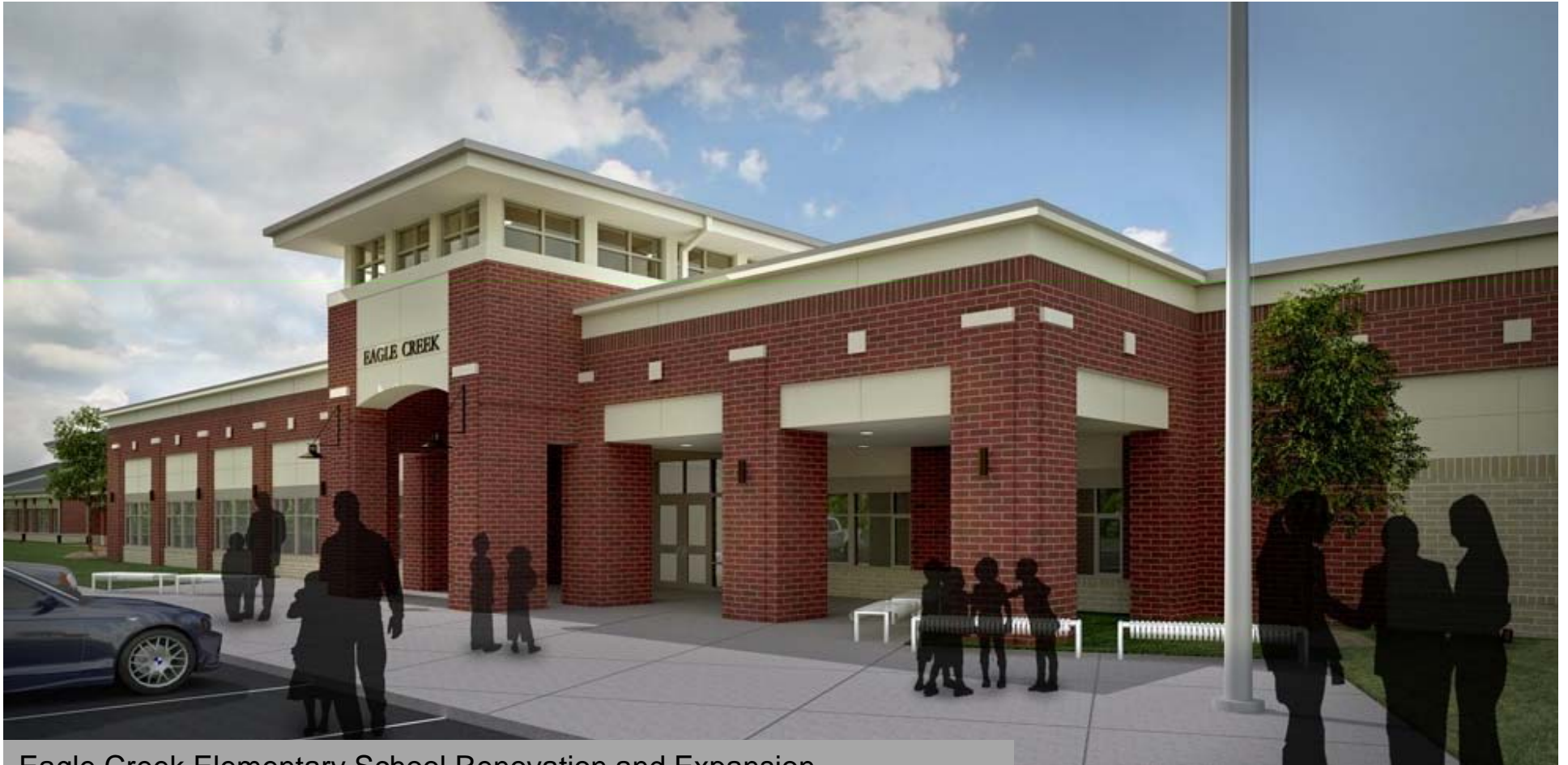
Eagle Creek Elementary School Renovation and Expansion
