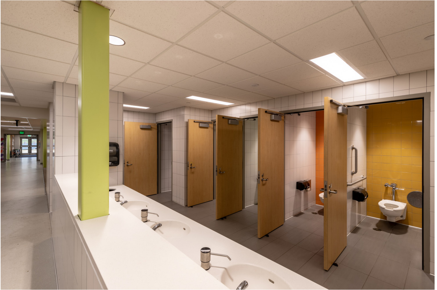
Figure 4: Inclusive restrooms are designed with full height acoustic partitions, photo of SPPS St. Anthony Park Elementary School.
