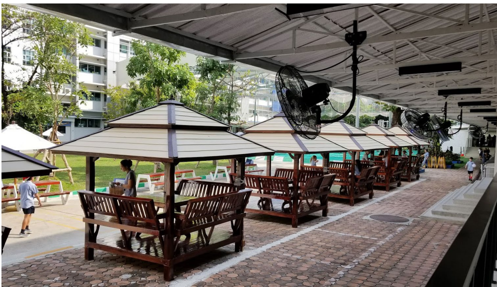
FIGURE 97. Outdoor spaces that may have been uninhabitable due to heat and humidity are used here to create family-style groupings of students in small gazebos. Fans keep the air moving and allow such spaces to be used all day long.
