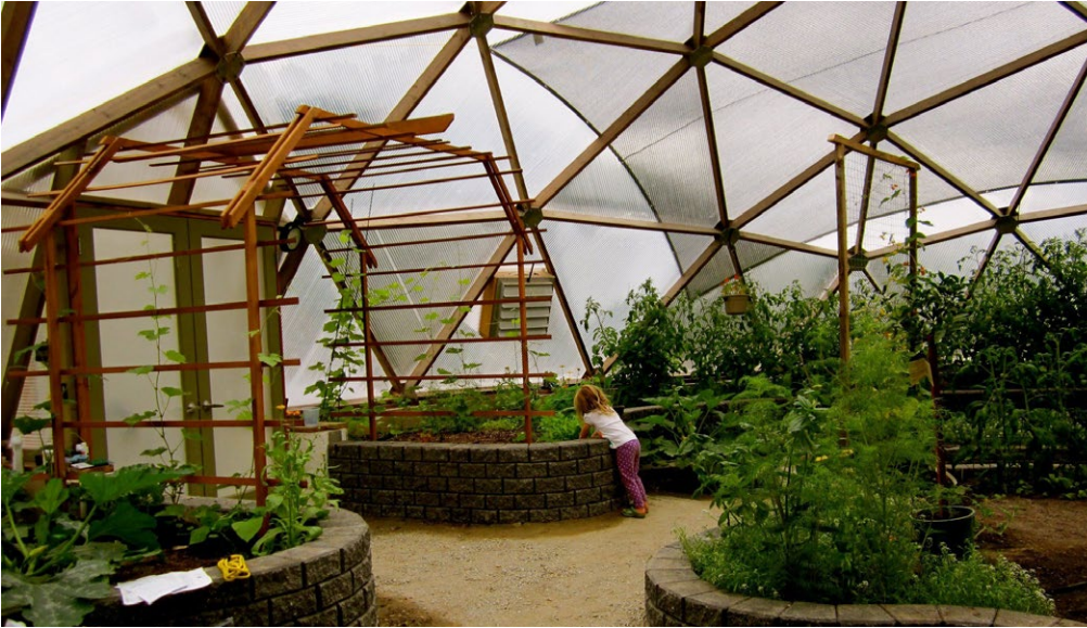
FIGURE 98. This is a greenhouse built as a geodesic dome in BC, Canada. It is a quick way to cover an area to make it habitable all year and a fun place for children to learn in. The geodesic dome itself is a fascinating engineering subject for study. Photo: Donna Hausken
