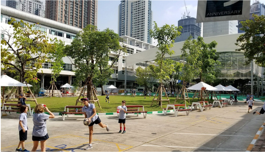
FIGURE 95. At NIST International School in Bangkok, Thailand, in the background a shade structure is visible that provides protection from driving winds and rain, which is important in a tropical country like Thailand.
