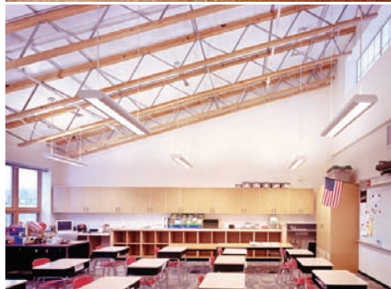
Clearview Elementary School John Boecker, Architect with L. Robert Kimball & Assoc. Photo: Jim Schafer Location Photography
